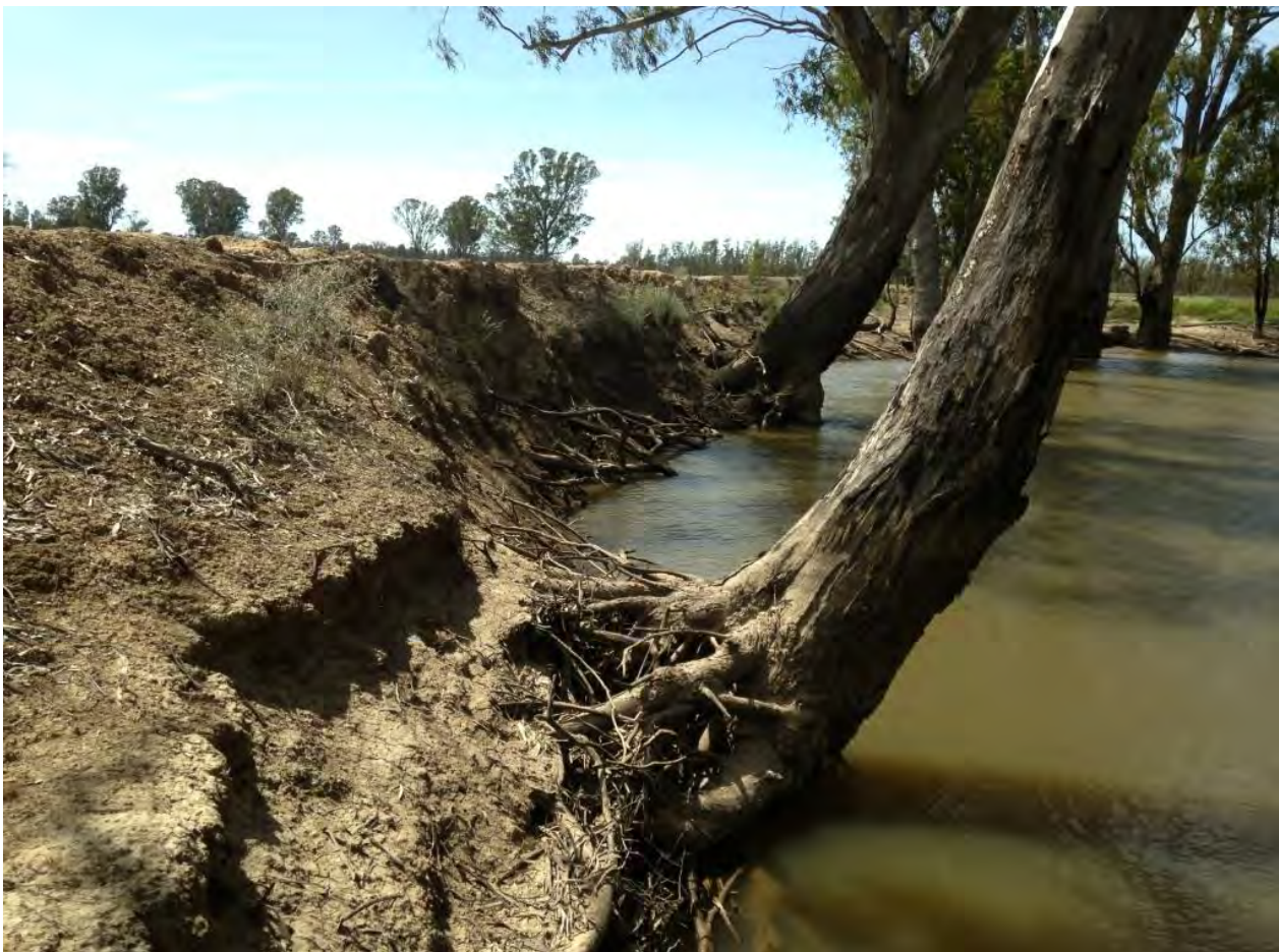
Levee bank within the reach showing erosion on the levee toe associated with tree growth. Photo: Terry Korodaj, MDBA.
