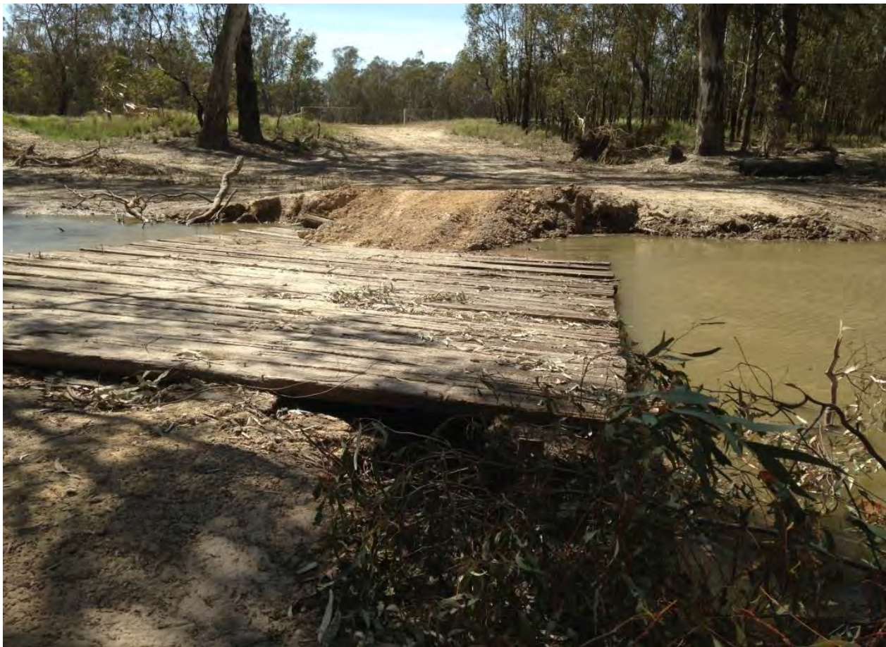
Repair works on a low-lying creek crossing following damage associated from an earlier natural flow event. Photo: Terry Korodaj, MDBA.
