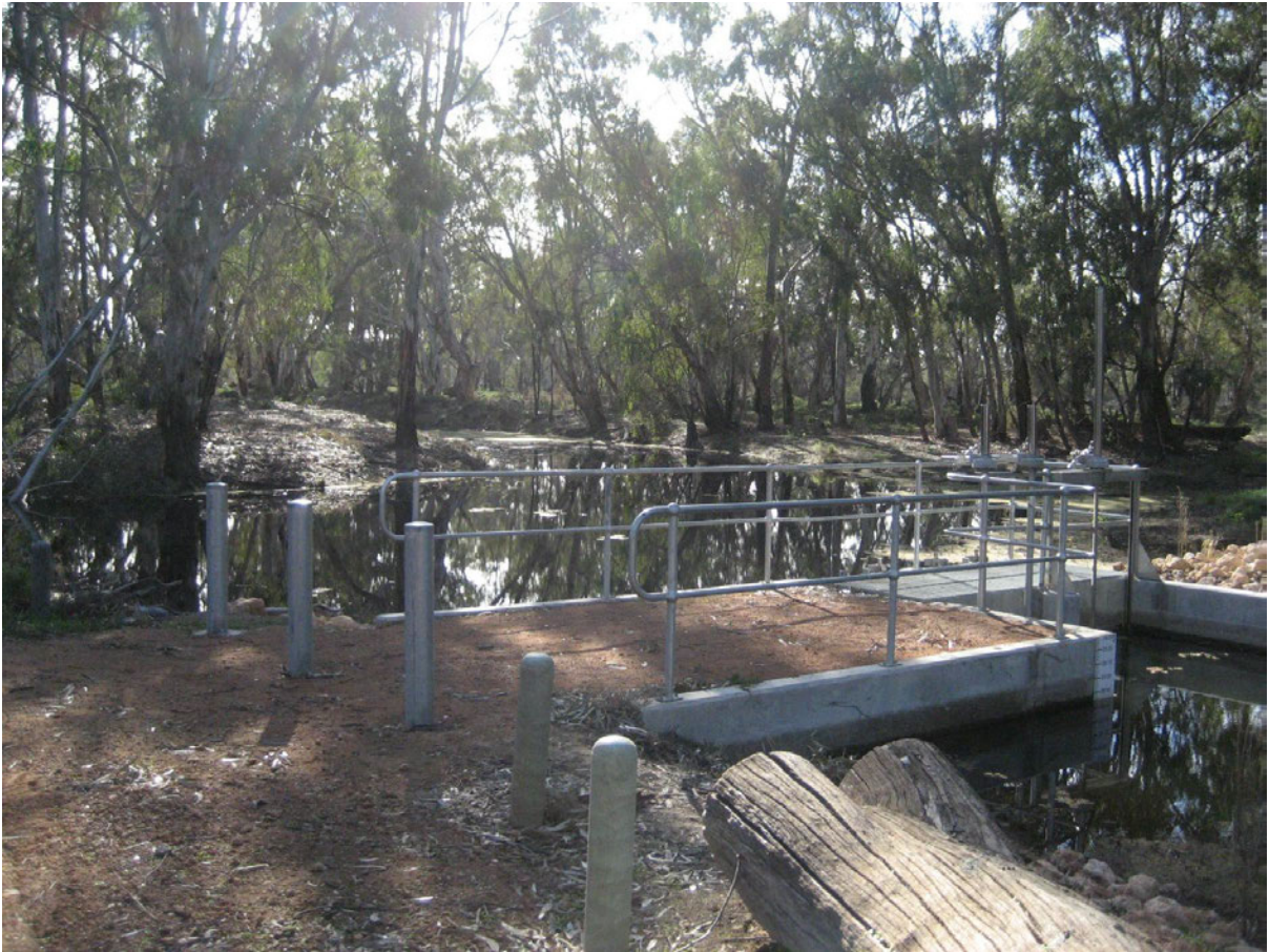
The Horseshoe Lagoon Regulator, Wallpolla Island, constructed under The Living Murray Program in 2006.
