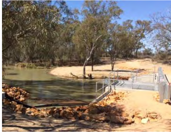
Figure 9: Eckert Creek Regulator and Fishway at Katfish Reach constructed as part of RRP at Eckert Creek ( Photo courtesy of H. Pocock, 2015 ).
