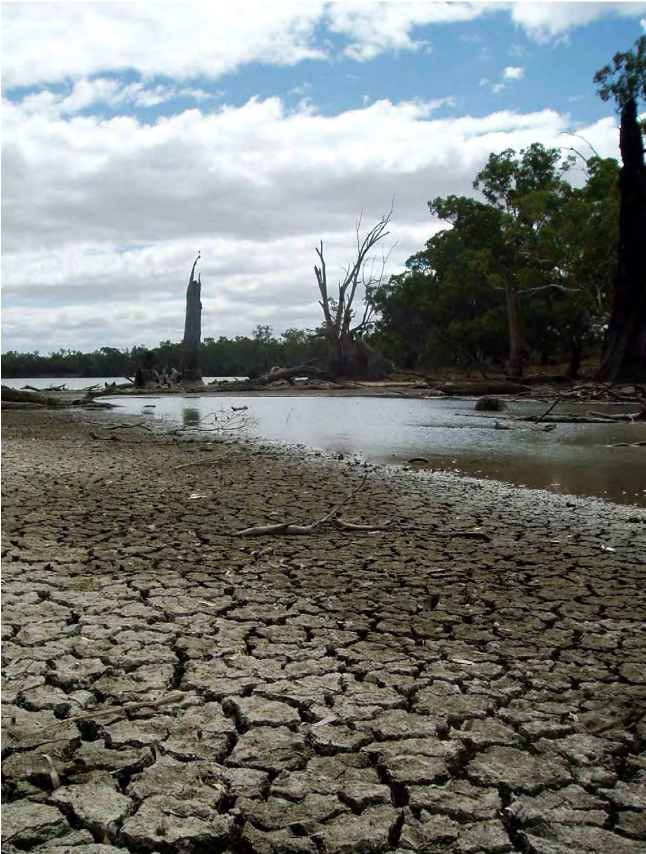
Figure 4-2: River Murray – Lock 8 weir pool drawdown event (left): exposure of dry silts for reconsolidation [Source S. Jaensch, April 2015]
