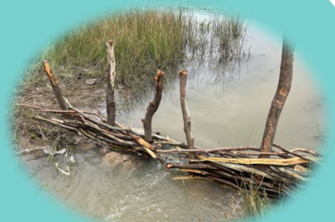
Indigenous weir constructed by the JIG crew in-situ at the Pollack Swamp (Source: Dan Hutton)
