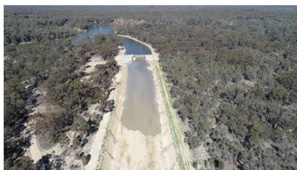
Water is measured as it flows into Koondrook-Perricoota Forest at the inlet flow regulator (Photo: NSW Forestry)
