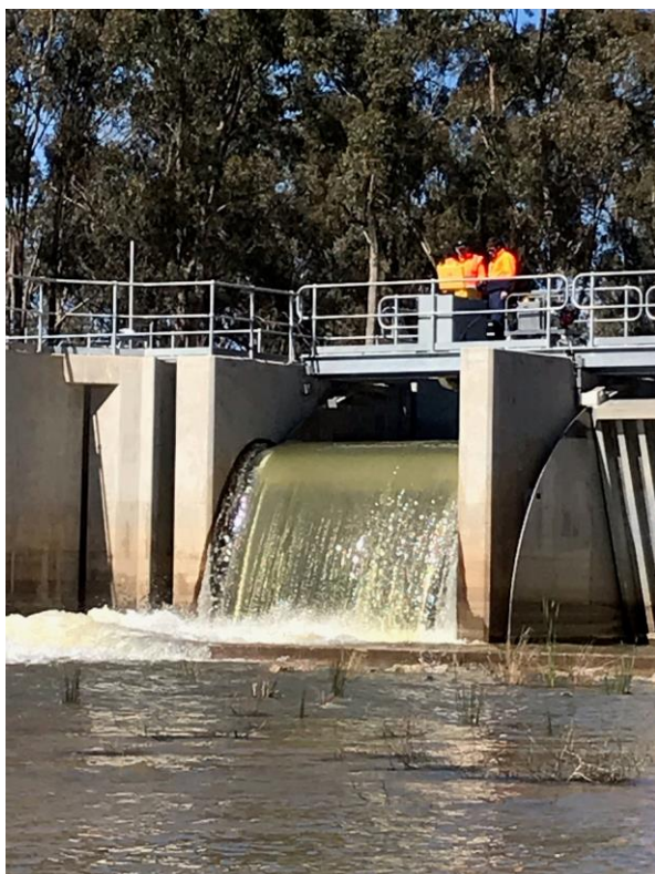
Water is measured as it flows into Koondrook-Perricoota Forest at the inlet flow regulator (Photo: NSW Forestry)
