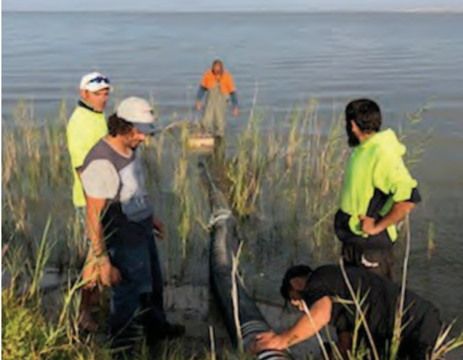
Raukkan working on Country rangers installing suction pipe into Lake Alexandrina, offtake point for Teringie Wetland filling (photo by S. Long)
