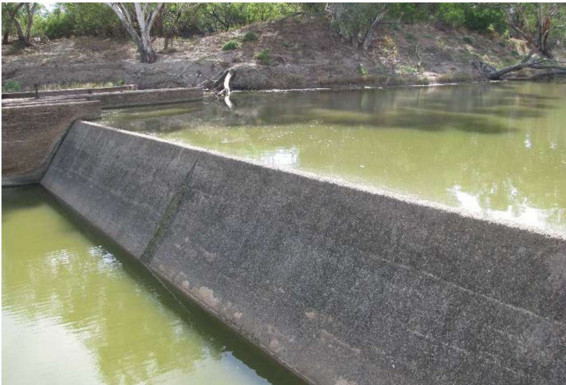
Figure 11: Bourke Weir on the Darling River: an example of significant barrier to fish passage on the Darling River (Photo: Adam Sluggett, April 2015)
