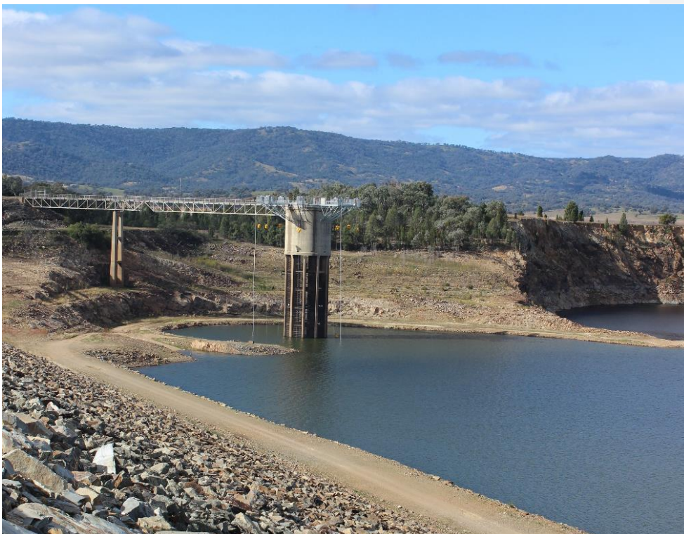
Figure 9 Burrendong Dam offtake tower with cold water curtain. Photo: Tim Hosking/OEH
