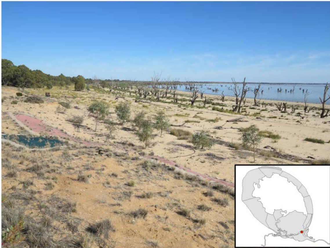
Figure 14 Snake Island foreshore with burial protection works in upper elevations and sand erosion control measures in lower elevations(2014) and location of photo (inset). Photo credit: Daniel Haines (SAW).
