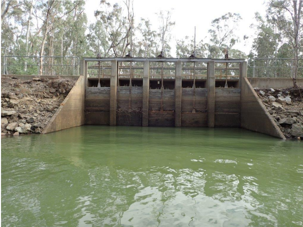
Figure 19. A regulator which controls flows into the Gulf Creek on the Victoria side of the Murray River, approximately 46 river kilometres upstream of Barmah Lake in 2016 (photo courtesy of Keith Ward, Goulburn Broken Catchment Management Authority).
