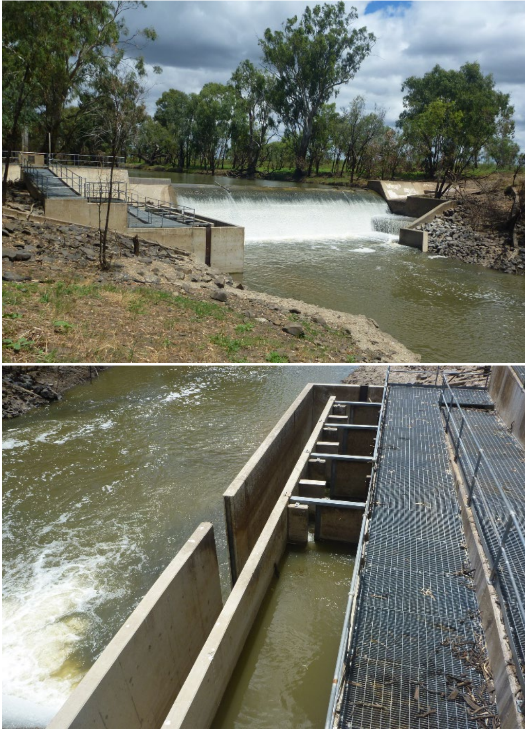
Figure 3. Above: Loudoun Weir on the Condamine River near Dalby with a vertical slot fishway on the left bank. Below: Detail of the fishway in operation (photos courtesy of Greg Ringwood, Murray–Darling Basin Authority).
