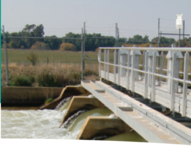
Left: Automated flume gates installed as part of a program to improve water efficiency in the Shepparton Irrigation District, Victoria.
