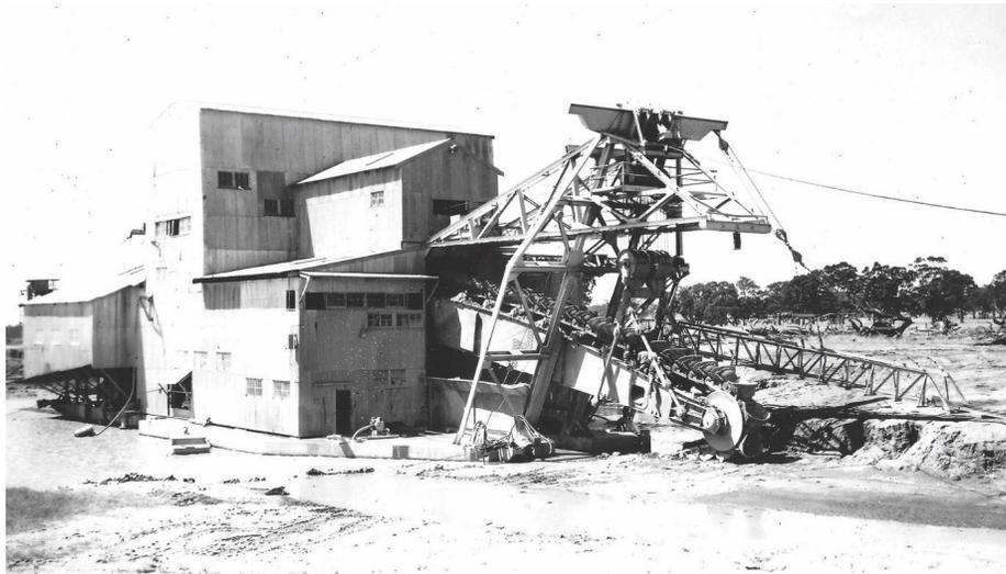
**Figure 7-12.** A photograph of the Newstead Dredge on the Loddon River floodplain showing the buckets at the front of the machine.
