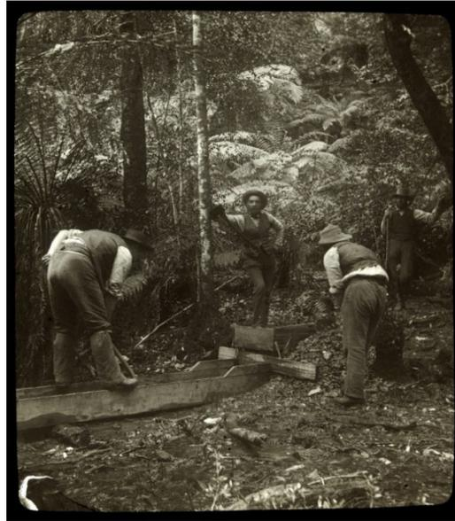
*Figure 7-5. Three men using a long tom and sluice box, ca. 1890 H2009.100/148 (photo courtesy of the State Library of Victoria).*
