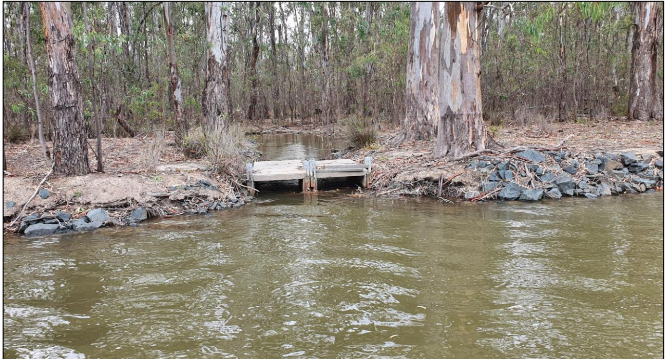
Figure 31 Example of existing bank protection works at a small regulating structure on the Barmah-Millewa reach upstream of the Edward River confluence. Image was captured by Professor Ian Rutherford in 2021.
