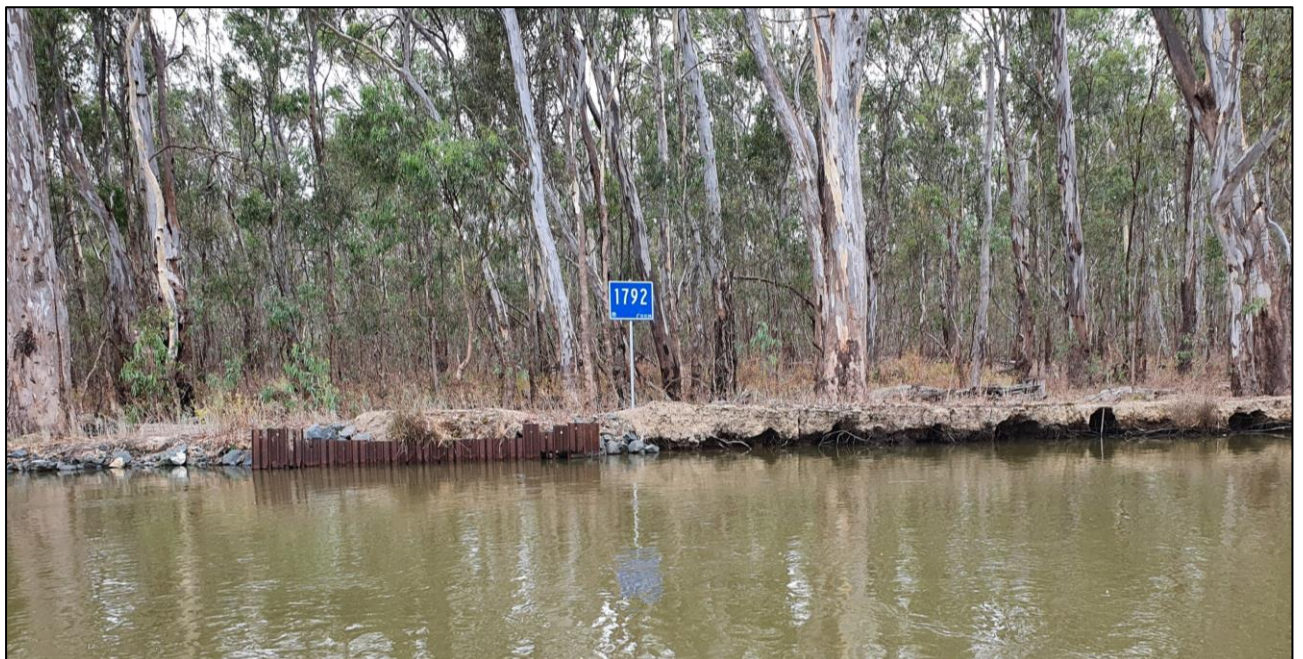
Figure 32 Example of existing bank protection works (sheet piling) on the Barmah-Millewa reach upstream of the Edward River confluence. Image was captured by Professor Ian Rutherford in 2021.
