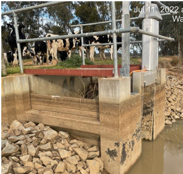
Discharge headwall (replace)
