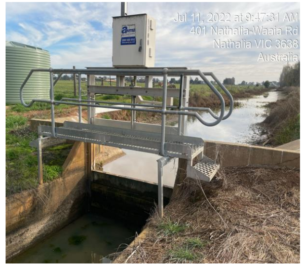
Discharge structure to creek (replace)
