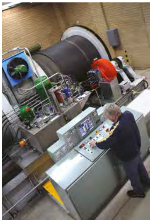
Dartmouth senior reservoir controller Peter Liepkalns demonstrating the newly completed low level outlet winch drive system. The winch raises and lowers the low level bulkhead, which weighs 25 tonnes. It is lowered to close off the reservoir's outlet tunnel so that inspections and maintenance can be carried out (photo by Andrew Beer, MDBA).
