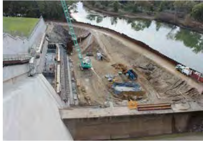
Hume Dam southern training wall buttress construction showing the completed upstream section (bottom left corner) and progress on the downstream mass concrete section (photo by Tony Morse, MDBA).
