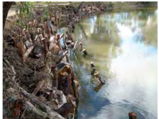
Log revetment is when logs are used to help protect river banks from erosion. Since 2007 it has become the most utilised technique for reducing erosion between Hume Dam and Lake Mulwala.
