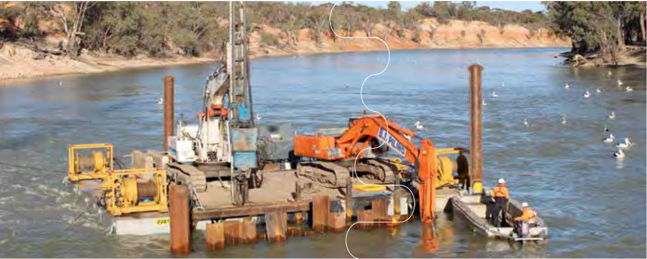
Driving sheet pile from a barge, downstream of Euston Weir and Lock 15. The works are to address downstream erosion as part of the overall Euston Weir upgrade (photo by Tony Morse, MDBA).
