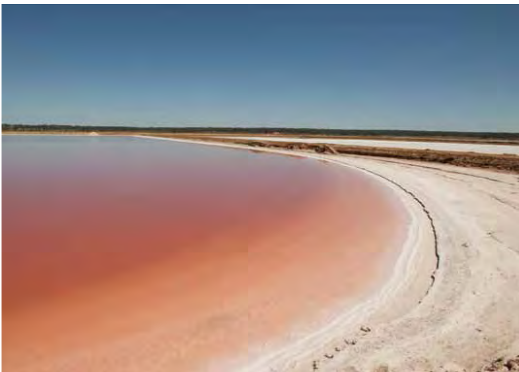
Evaporation ponds, Buronga groundwater salt interception scheme, NSW. Salt from the evaporation ponds is harvested by Mildura company SunSalt, and is exported all over the world.
