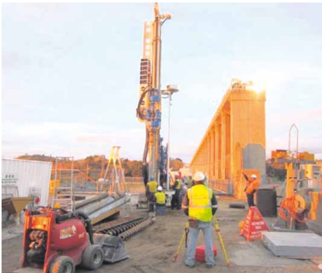
Drilling work in progress at Hume Dam for the installation of an improved filter and drainage system at the spillway southern junction
