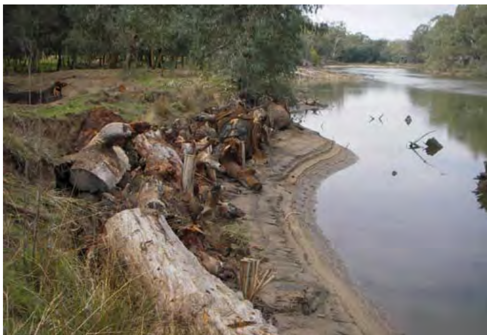
Controlling erosion with a log revetment on the River Murray near Corowa
