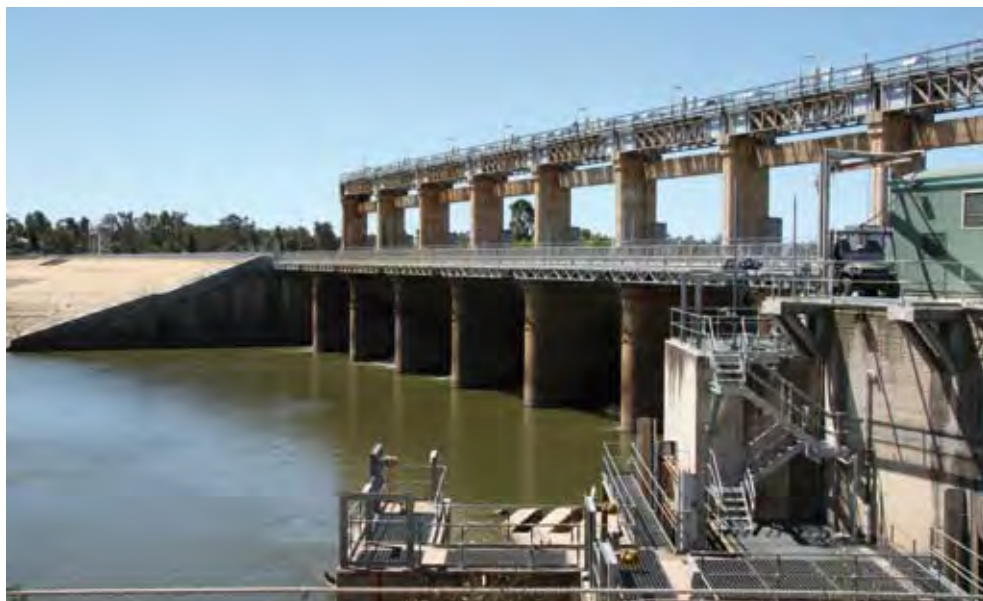
View from downstream of Yarrawonga Weir showing the southern structure gates, superstructure housing the winches, and the fish lock adjacent to the power station in the foreground.
