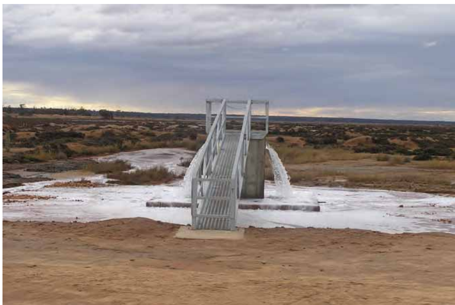
Outfall structure for the Buronga Salt Interception Scheme
