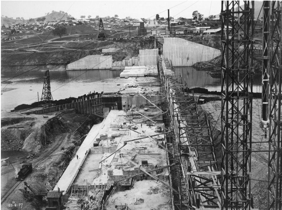
Construction of Hume Dam—work proceeding inside Cofferdam, 25 August 1927 (see page 59)
