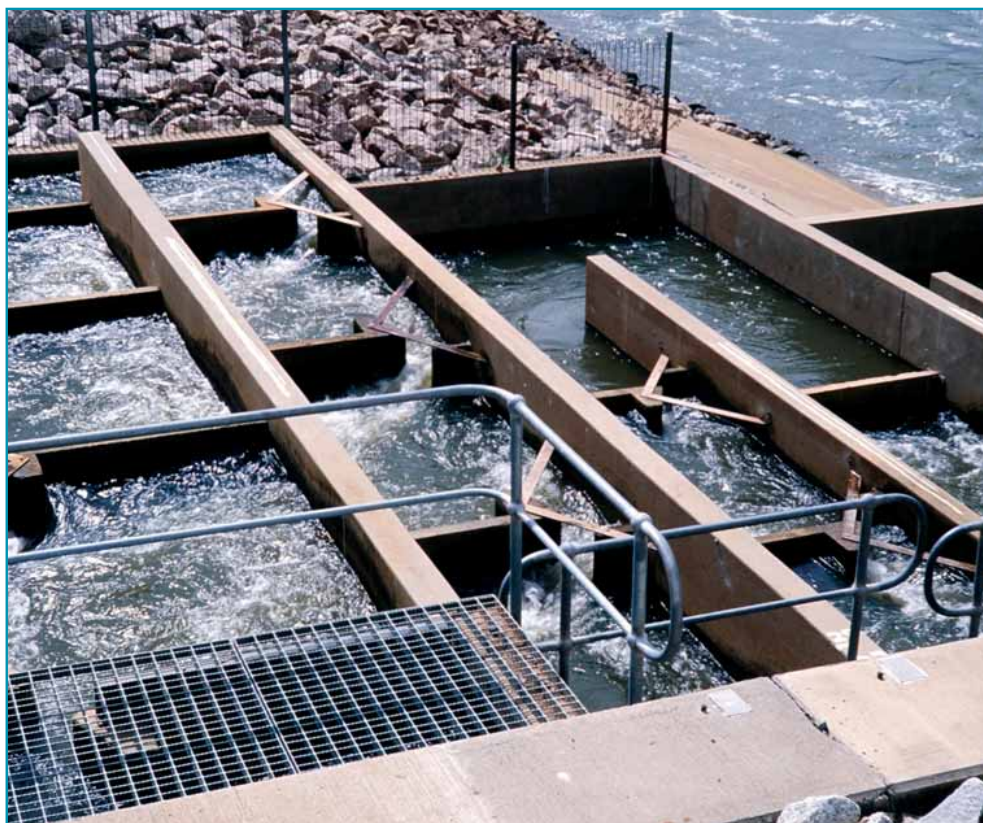
Vertical slot fishway
