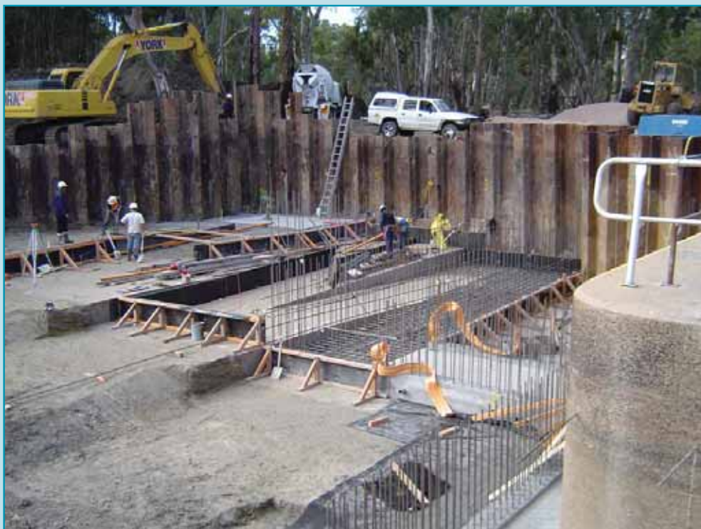
Vertical-slot fishway under construction at Lock 8, River Murray
